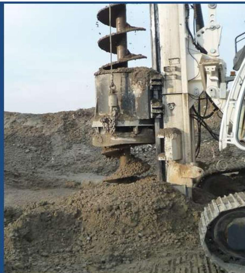
Trevi machineries at work for extracting the gravel and replacing it with cement grout
