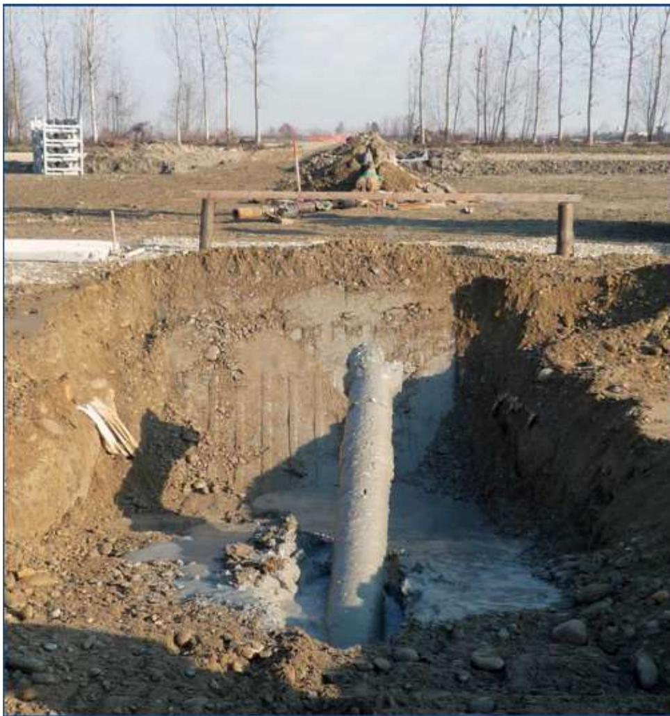
Punching out of the drilling string, perfectly aligned with the product pipe string
